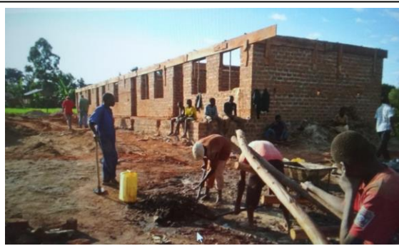
Construction underway on the classroom block
