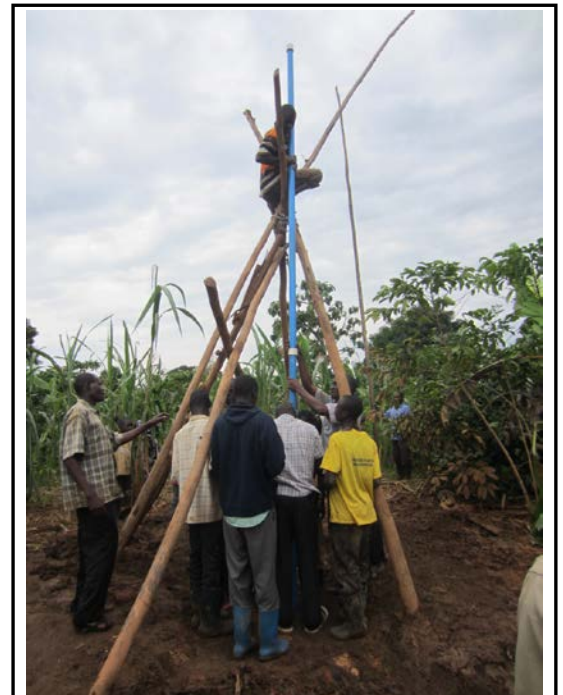
Children in Buyaga Village are assigned to haul water in jerrycans from a contaminated open water source located a quarter of a mile away. The young men from the village were taught a method for manually drilling a well.
